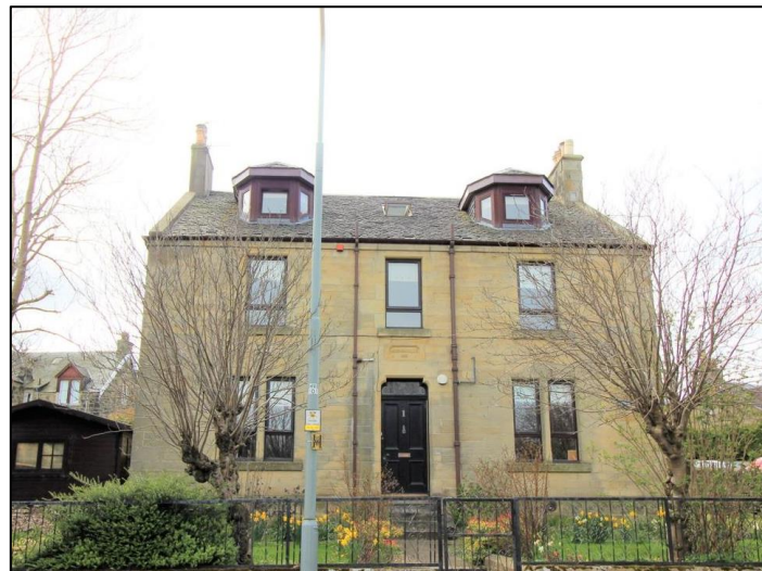
1, Harburn Road, West Calder
